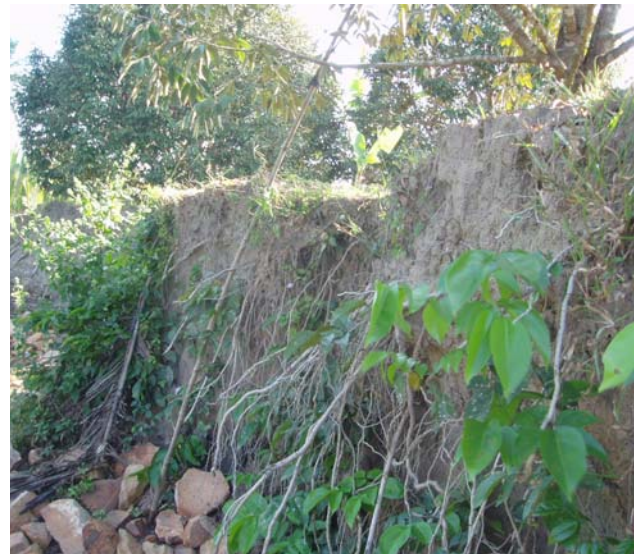
Exposed roots on the riverbank are evidence of erosion caused by sand-pumping, which threatens farmers' livelihoods.
